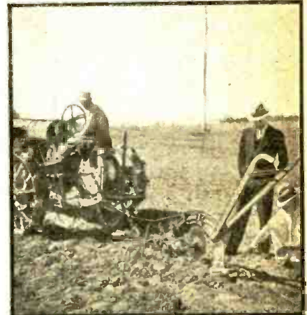
Laying 50 miles of copper wire which is an unseen factor in the efficiency of the new KDKA antenna; it is buried about a foot deep, to form a ground. In the background, masts of KDKA's multiple system.
